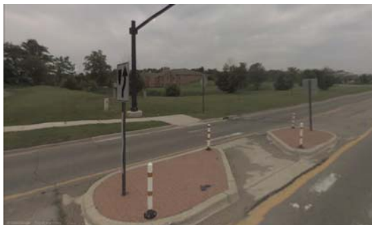
Oak Valley Road, Pittsfield Township (Google Street View)
