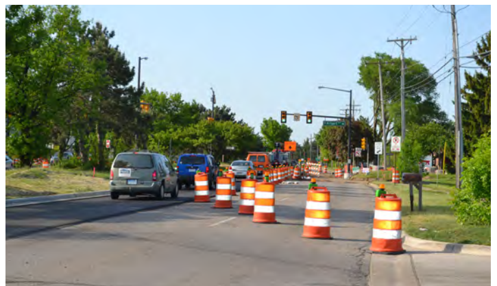
Intersections such as Research Park Drive and State Street need signal, signage, and pattern improvements
