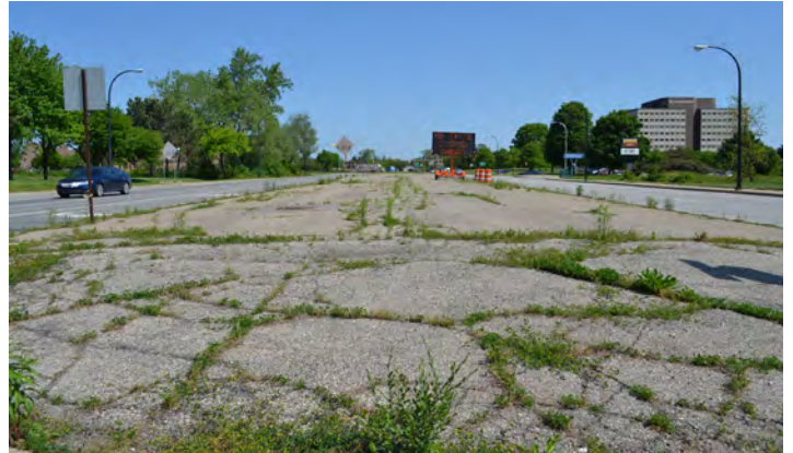
Concrete medians dominate the landscape in Area 2
